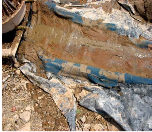
Fig. 4.6 - Clogged trapping mechanism (blanket) of hand-fed sluice
