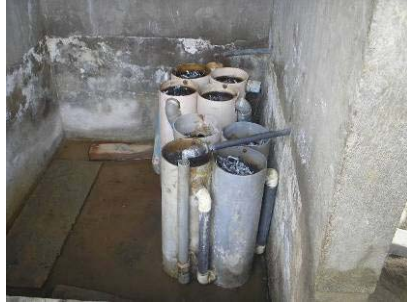
Fig. 6.7 - PVC Columns used for gold precipitation with zinc shavings
